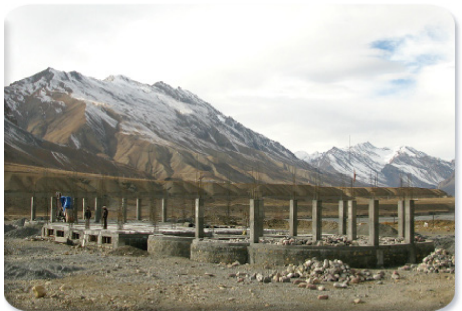
Construction has begun and the foundation has been laid
